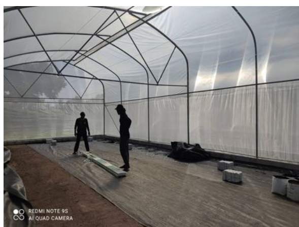
Picture 3: Leveling the ground and putting the weed mat
