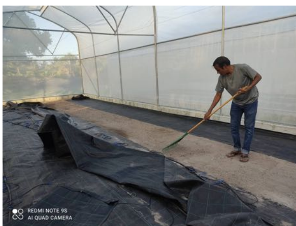
Picture 4: Leveling the ground and putting the weed mat
