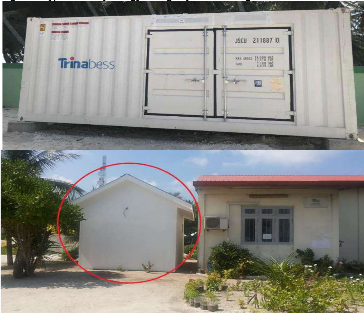
Top image: containerized BESS system; Bottom image: BESS building Source: MOECCT
