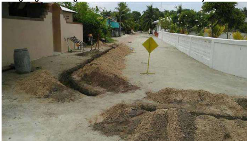
Figure 19: Ongoing Trenching for Cable Work under POISED Project in Goidhoo Island
